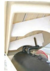
Cover can be lifted to check tank gauge after installing external fill and vent.
